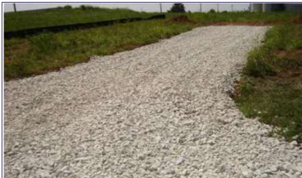
Figure 8.1: Temporary access track
